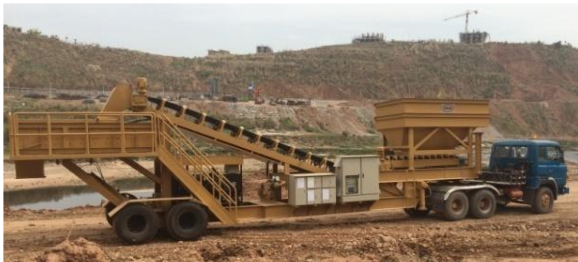
A FOAR MOBILE PUGMILL PLANT AT A CLIENT'S PROJECT SITE
